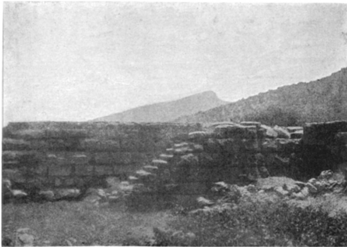
FIG. 13.—WALL FROM INSIDE SHOWING STAIRS AND GATE, NISYROS.
